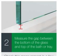
Check this measurement in a few different places, as the gap can sometimes vary in size.
